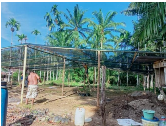
Figure 8. The construction of a 10 × 10 meters nursery in Ujung Bandar Village.
