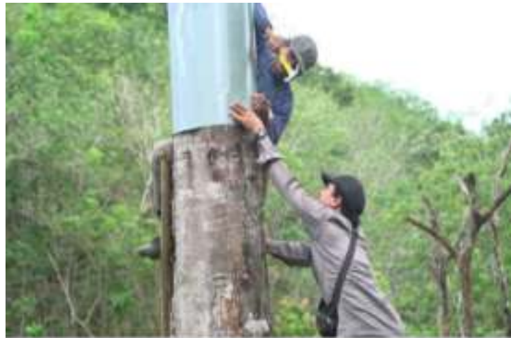
Picture 33. Zink plate installation in Batu Jongjong Village
