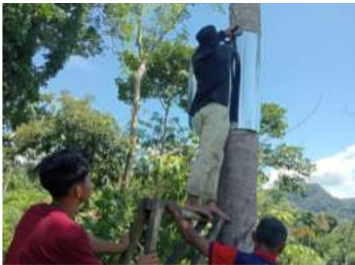
Picture 34. Zink plate installation in Lau Damak Village
